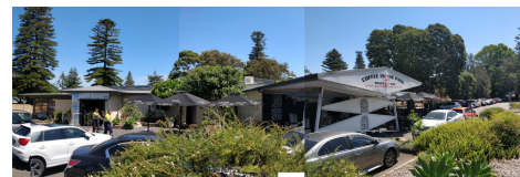
Figure 2f: Existing building viewed from Russell Avenue
